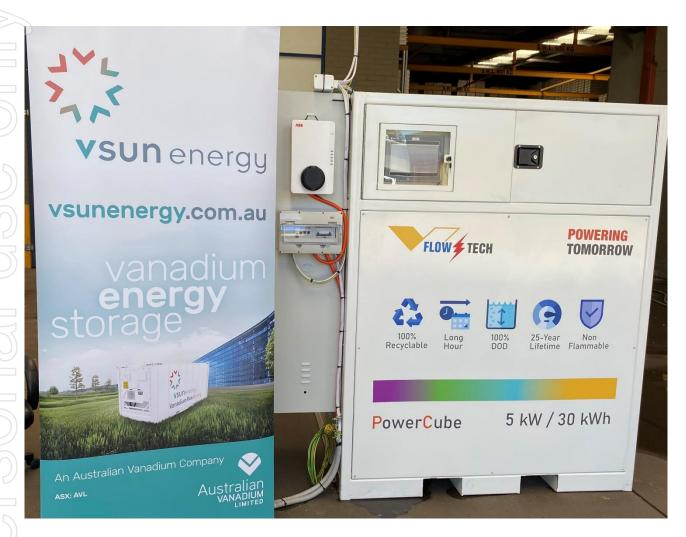
Figure 1 VRFB with EV charger installed
